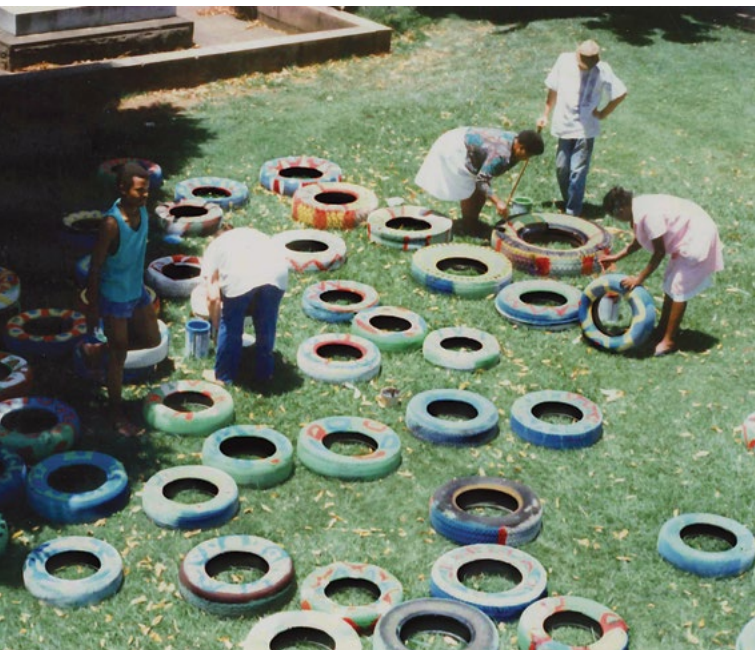
Laying out colourfully painted tyres in the Pietermaritzburg city centre site where The Peace Tree will be built. Photo: Zak Benjamin.
